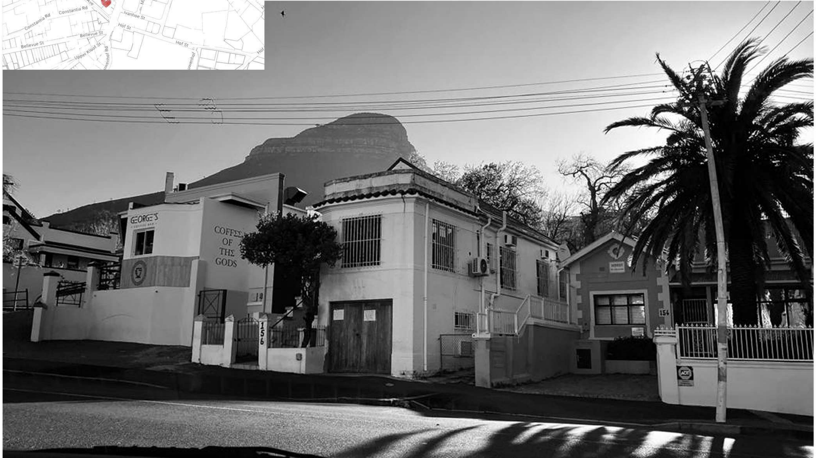
CURRENT LOCATION PHOTOGRAHED
