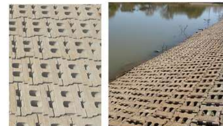
ARMOFLEX BLOCKS IN DAM RESTORATION ASSISTING WITH SOIL EROSION, DRAINAGE AND FILTRATION
