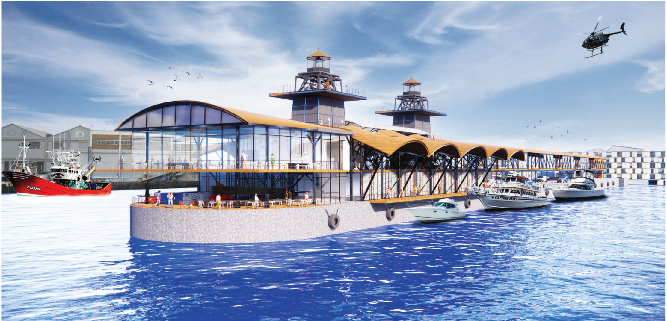
^ COLLIER JETTY FACADE
